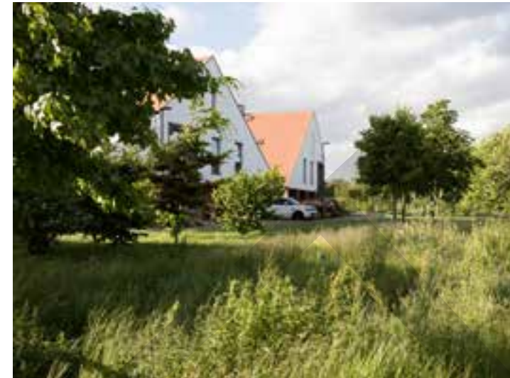
Medium density housing facing onto POS in 'Royston Green'
