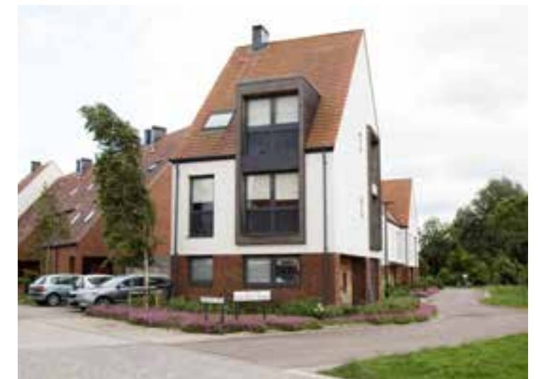
Derwenthorpe, York, where houses are designed to comply with the requirements of Lifetime Homes
