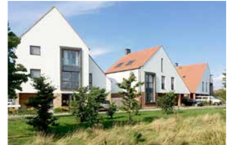
Homes - Well designed modern homes should be well integrated with open space and nature
