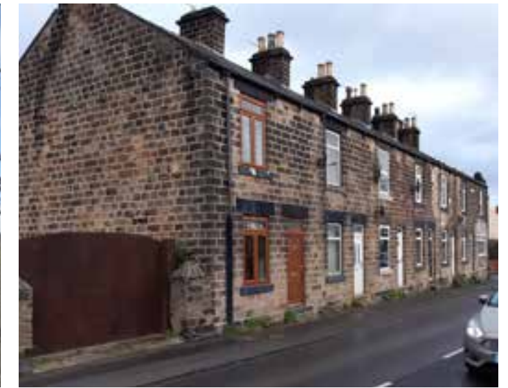
Existing terraced housing along Lee Lane consisting of sandstone and slate roofs
