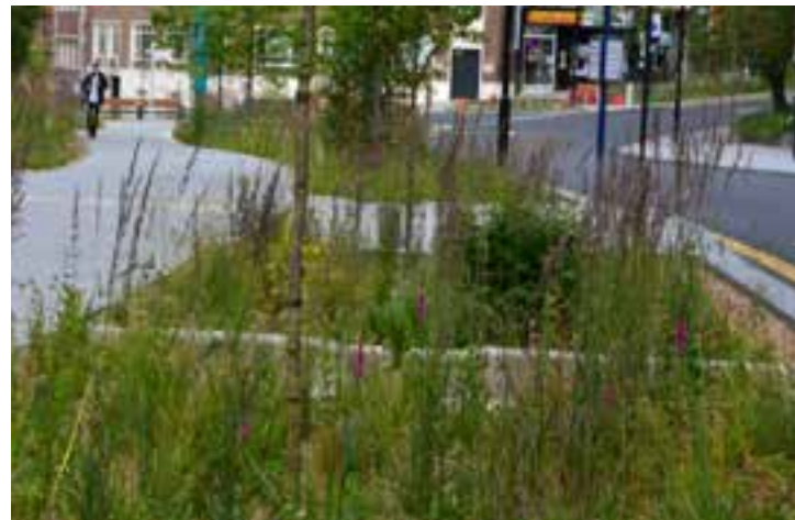
Sunken planters as rain garden as part of SuDS
