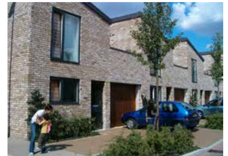
Example of dwellings with well designed integral parking space
