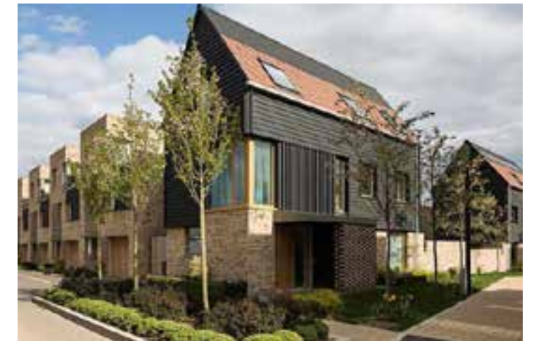
Precedent of well designed corner typology in residential plot. It is taller, dual aspect and has a more distinctive presence
